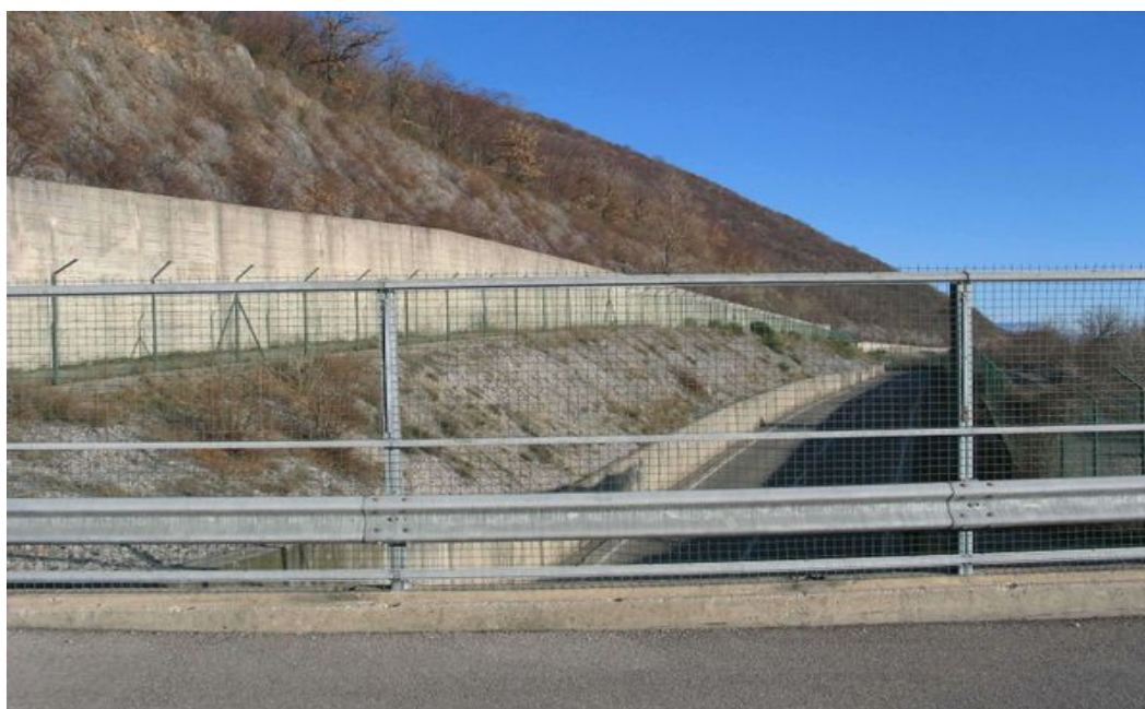
Figure 24 Road Bridge Over the Former Road Corridor Through the Italian Territory
