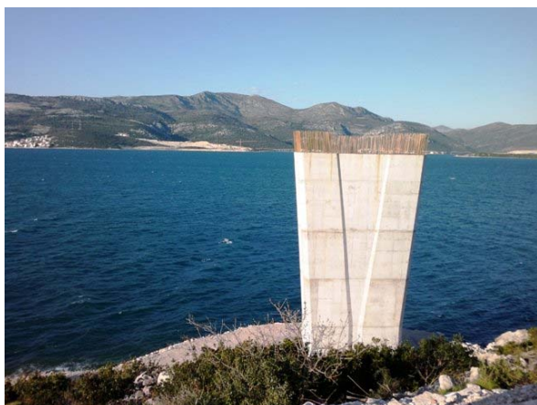
Figure 5 The Built Pillar of the Peljesac Bridge
