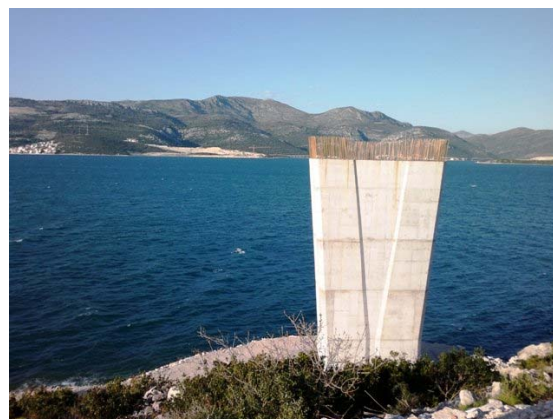
Figure 12 A Portion of Built Peljesac Bridge to be Dismantled to Build the Tunnel
